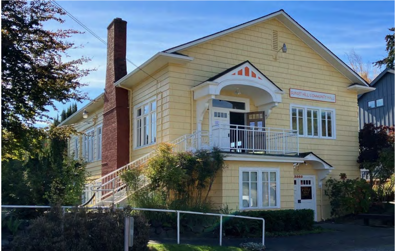
Figure 10: Primary (north) and secondary (east) elevations.
