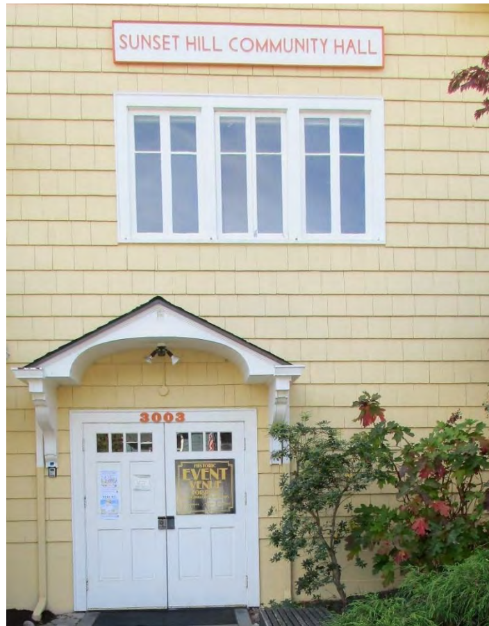
Figure 17: North elevation sign, window and ground floor (secondary) entrance, detail.
