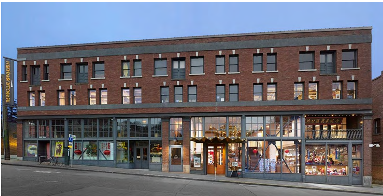
Figure 40: East Kong Yick Building (1910), Chinatown / International District Historic District. Lara Swimmer photo.
