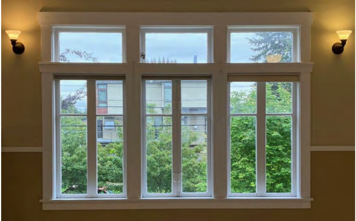
Figure 20: Main hall, east wall window detail.
