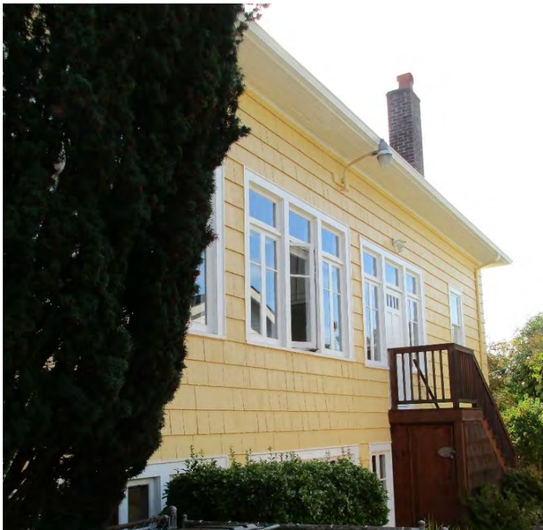
Figure 13: West elevation (note open window).
