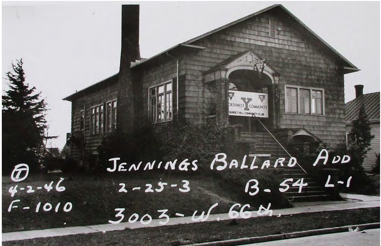
Figure 33: Property Record Card, 1946, shows roof reconstruction after 1944 fire. Puget Sound Regional Archives.
